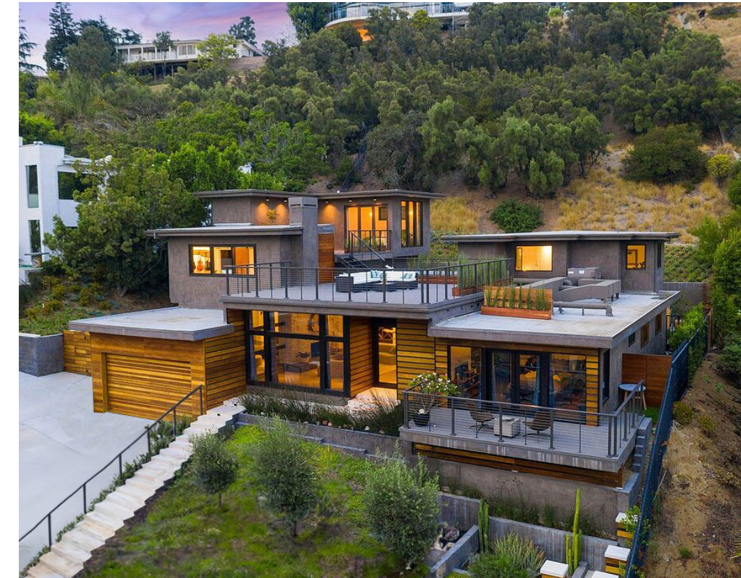
RESIDENCE STEP WITH EXISTING GRADE AND ROOF DECK
